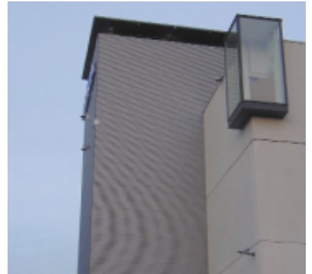
Ernitec housings and domes on the side/corner of the building.
